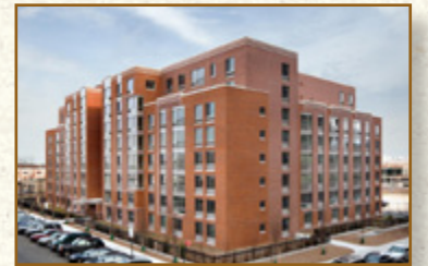
When completed, Dumont Green, located in the heart of East New York, Brooklyn, boasted the largest residential solar array in the State of New York.
