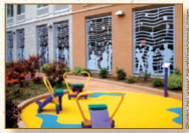
Built in partnership with the City and Habitat-NYC, Blue Sea Development's LEED Platinum Melody has made homeownership a reality for 63 low- and moderate-income families.
