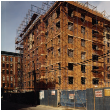
PALACIO DEL SOL 760 Melrose Avenue & East 156th Street Bronx, 110 Units (LAMP)
