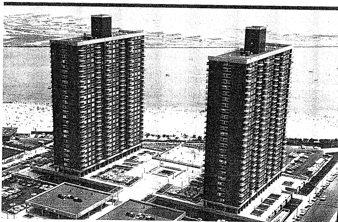
Ocean Park, an oceanfront moderate-income development located in Far Rockaway, Queens, is subsidized with Section 236 interest reduction subsidy funds.
