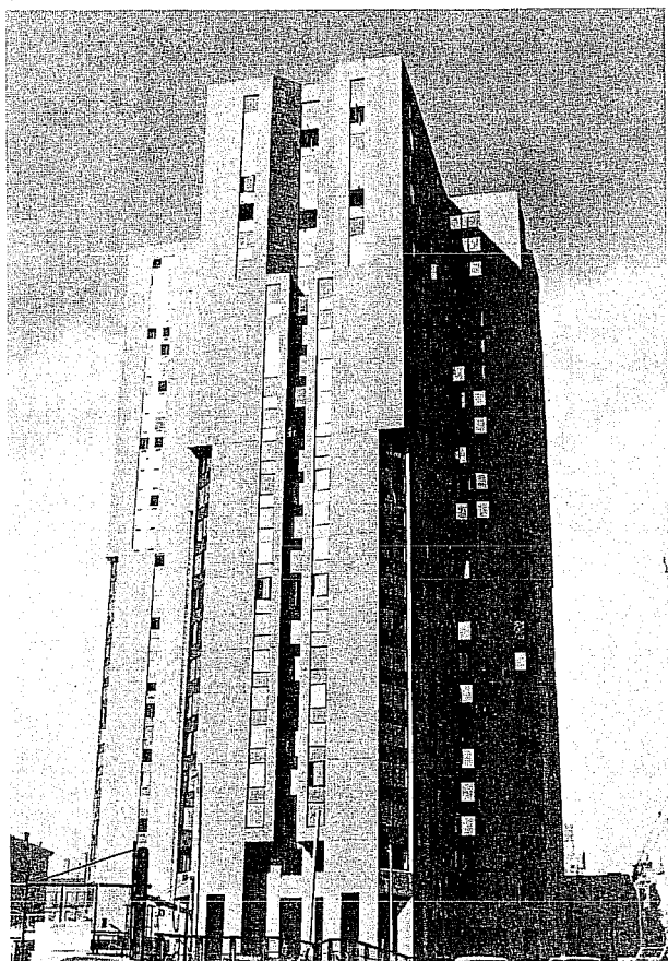
The Ruppert Towers Project (in construction)
