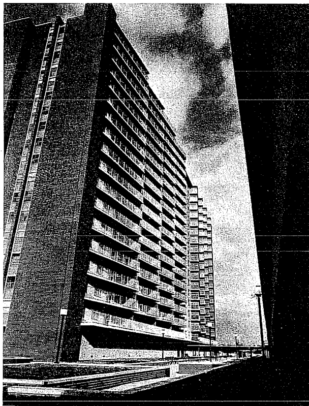
The Linden Plaza Project (completed)
